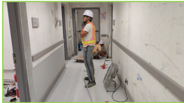
MTR Shatin Central Link In Progress
